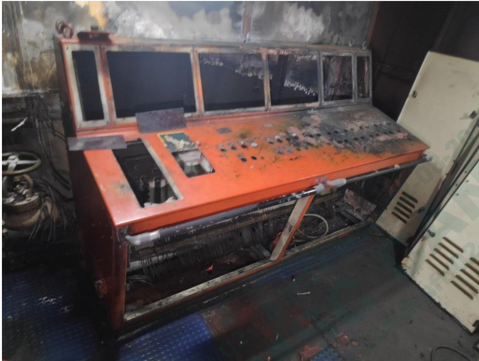
Main Control Panel totally burned.
