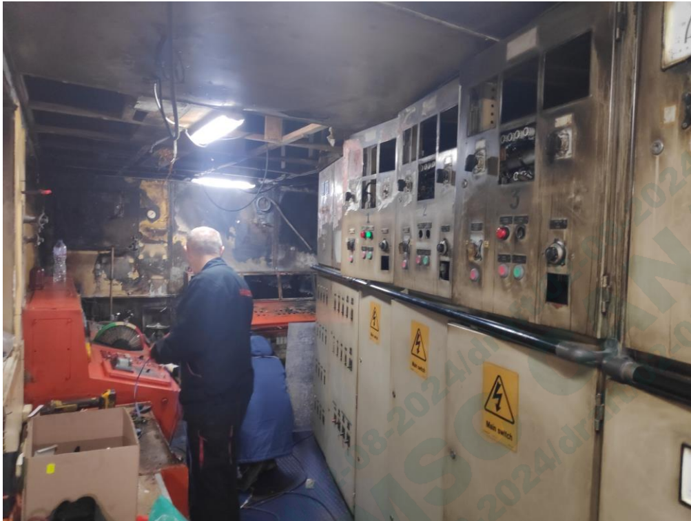
Control Panels partly burned.
