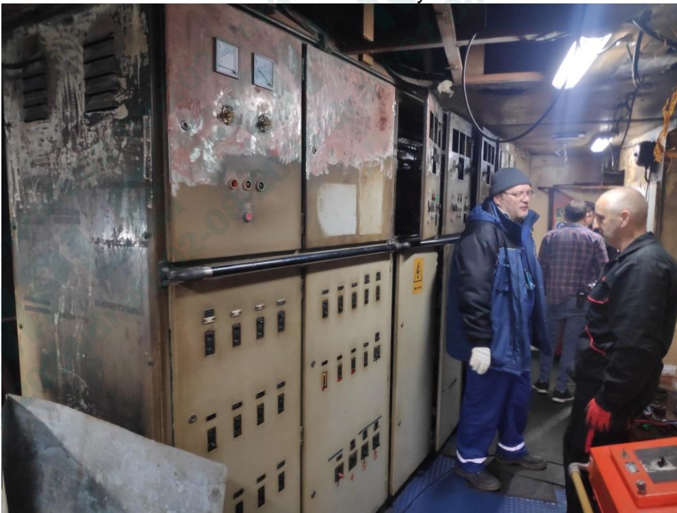
Control Panels partly burned.
