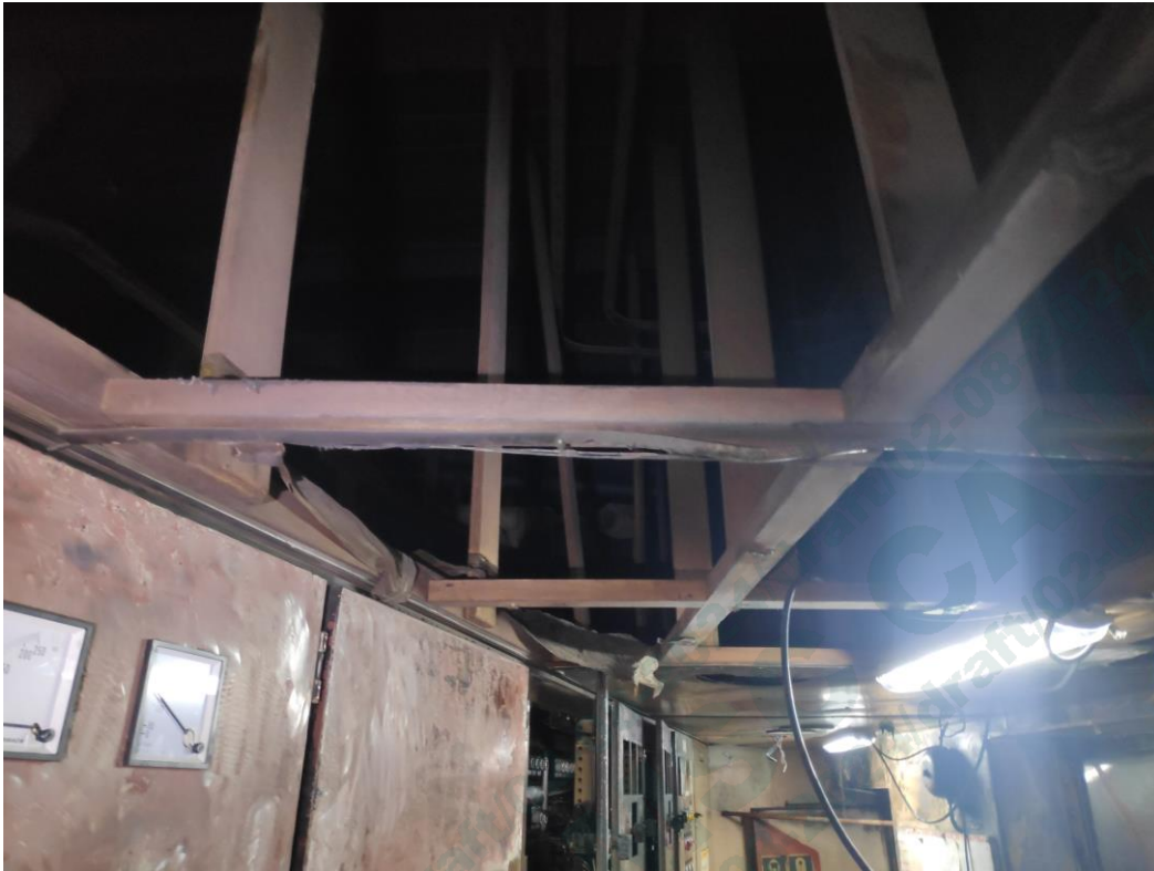
Ceiling totally burned and removed.
