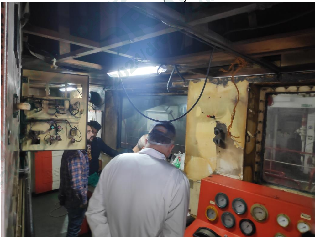
Ceiling totally burned and removed. Walls and floor partly burned.
